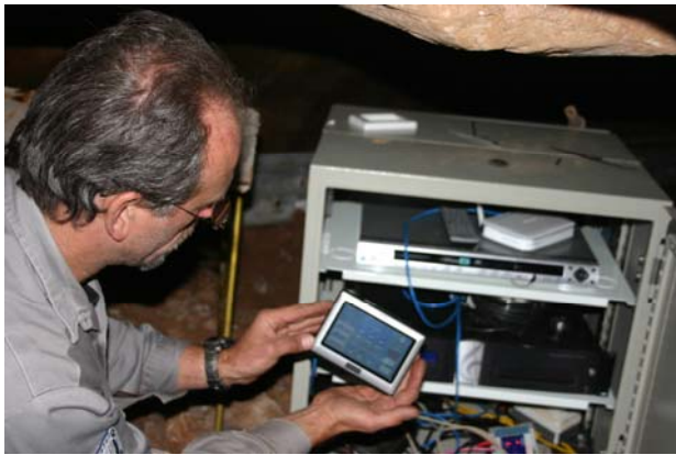
Dave Rowling with the digital control pad for The Temple of Baal – the entire lighting of the cave is controlled from this point.
